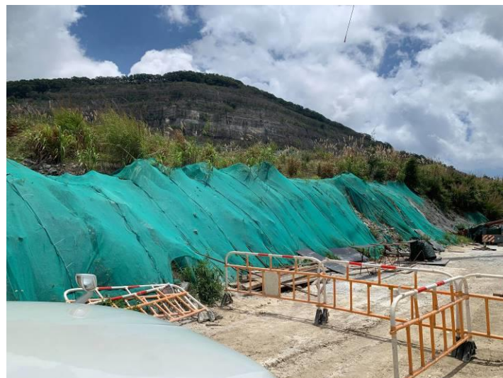
Impermeable cover for slope at System A.
